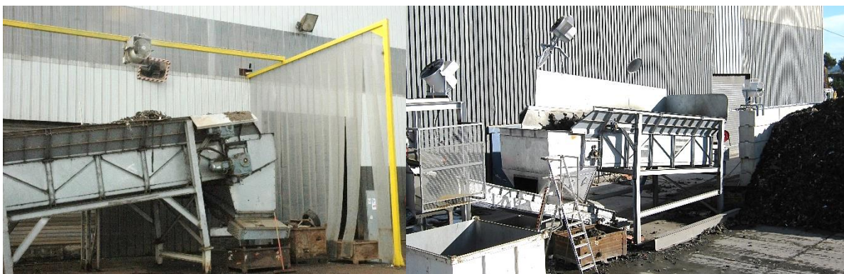
Waste treatment plant
